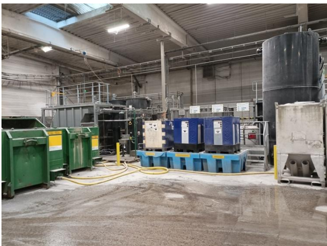
Figure 25 Left: Process water cleaning system and reagents used to in the process. Right: sludge which is mainly the mineral impurity removed from the waste stream.
