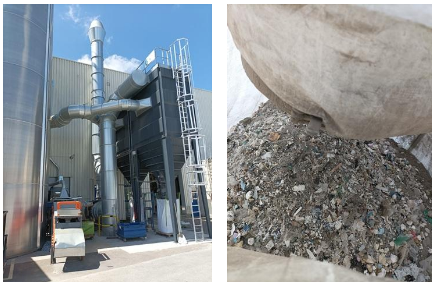
Figure 4 Left: Air Extraction Cleaning System with particulate filters. Right: Captured particulate matter.
