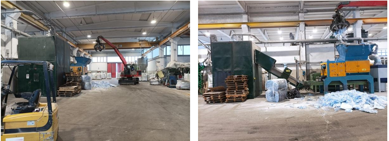
Figure 5 Mechanical Processing Hall. Left: crane used to feed the shredding equipment (blue machine). Right: Shredder being fed by pre-consumer foil and the subsequent grinding equipment (green boxed machine).
